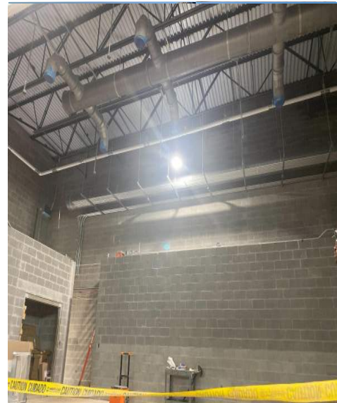
Ductwork installed in gym Area
